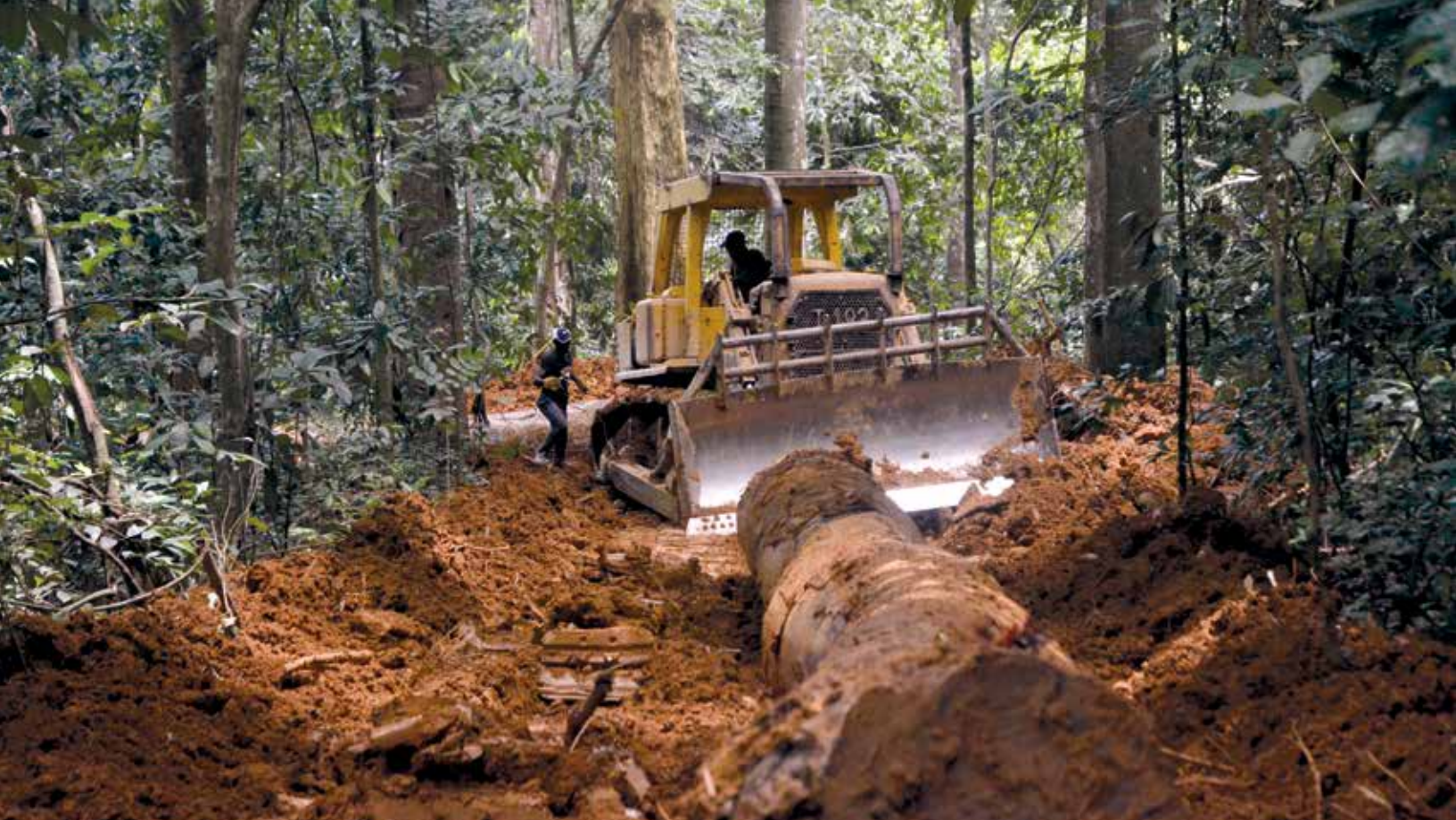
A bulldozer opening a secondary logging road in a forest concession in Gabon. Source: ANPN
