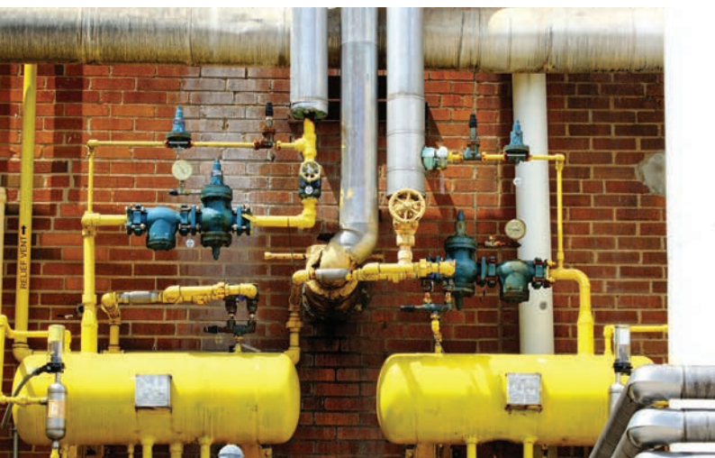
Above: Ammonia refrigeration tanks.
