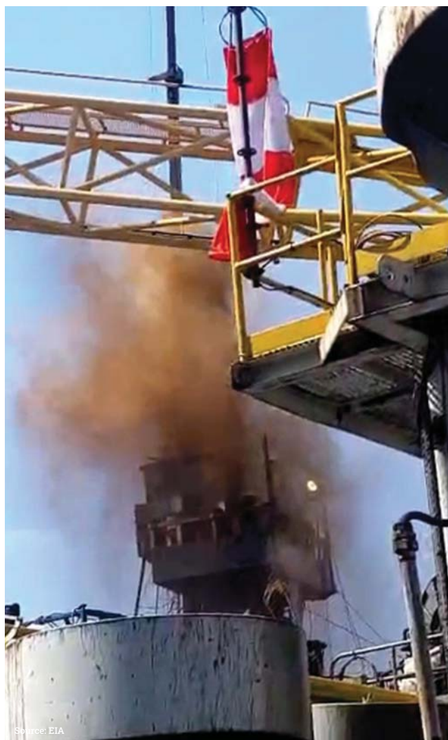
Figure 11 Oil surge that immediately preceded the fire on the Becuna platform, March 20, 2024.
