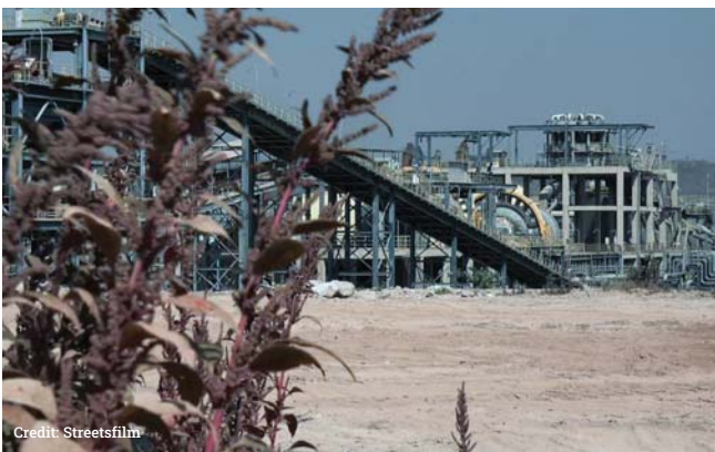
Figure 7 TFM's copper-cobalt processing facility
